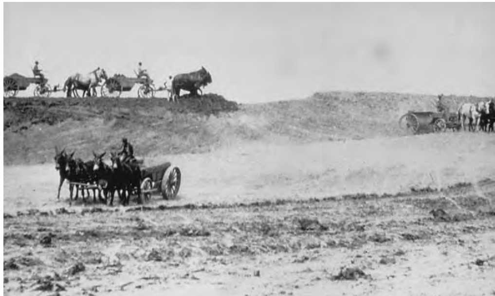
Early levee construction
