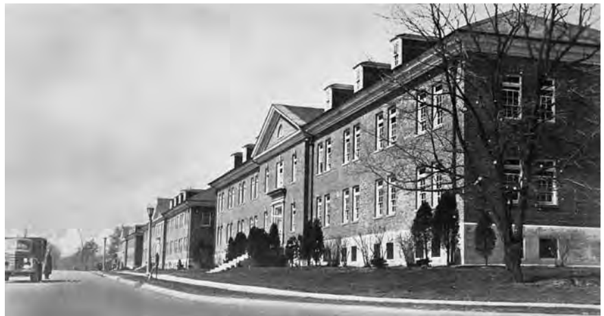
Company barracks, Fort Belvoir, Va., home of the U.S. Army Engineer School until 1988.
