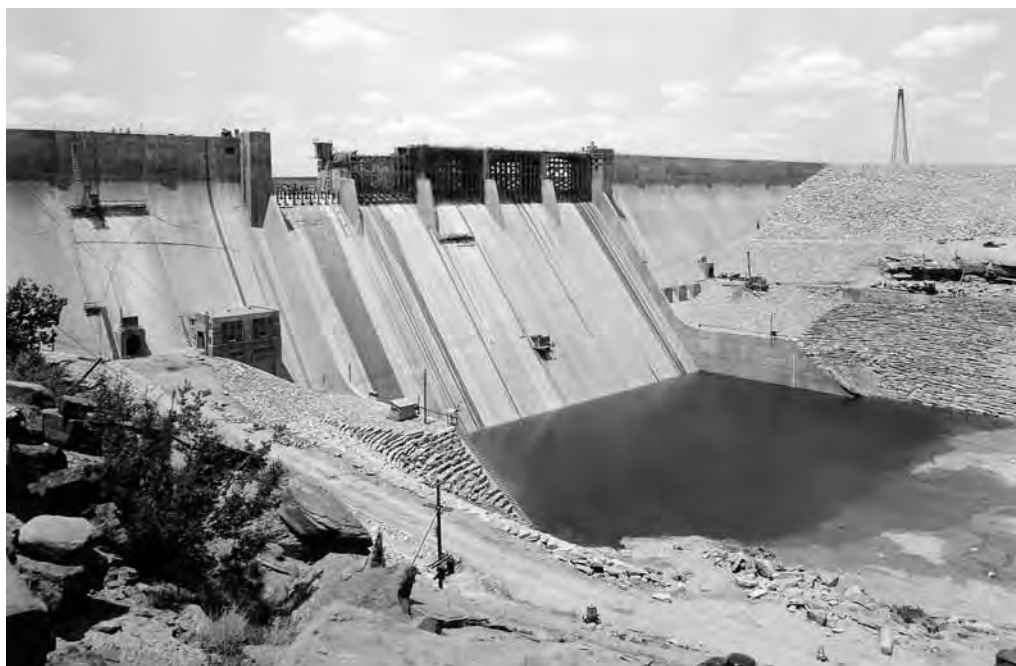
Construction of the Conchas Dam in northeast N.M., 1939
