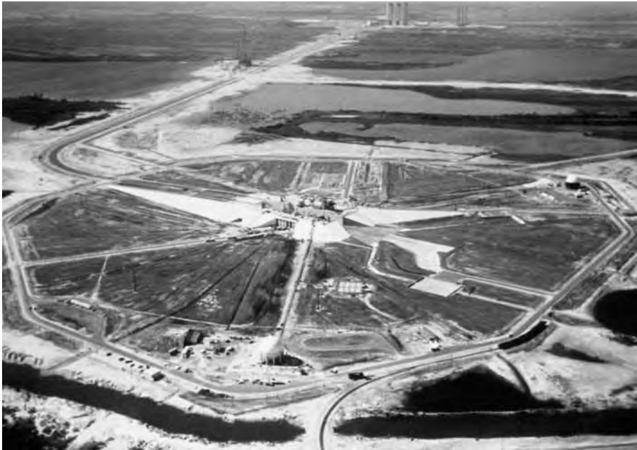
Launch Complex 39, Pad A, with the crawlerway connecting the pad to the Vehicle Assembly Building in the distance.
