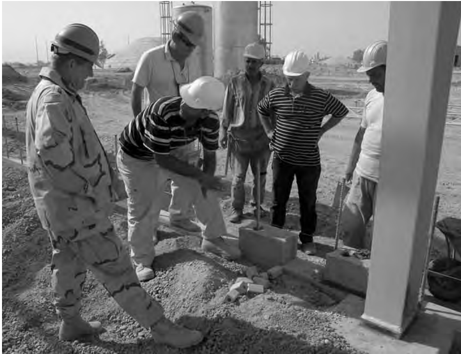
Engineers inspect the construction at logistics support area (LSA) Anaconda, July 2005
