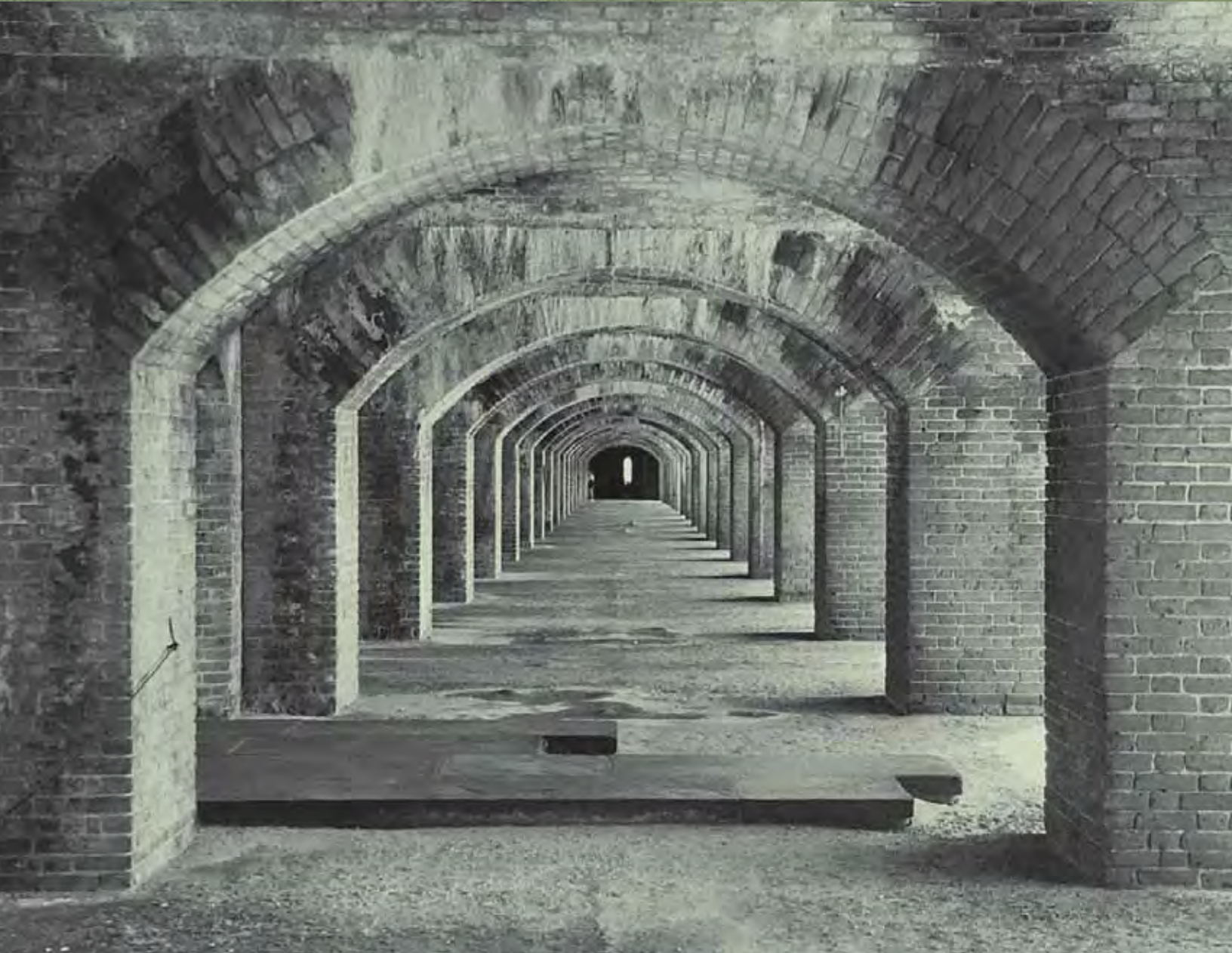
Interior view of the casemates at Fort Jefferson, Fla.
