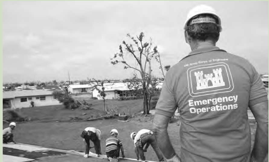
Corps and contractor personnel install temporary roofing, Perrine, Fla.
