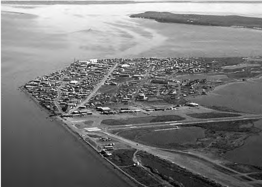
Kotzebue, a hub village in northwestern Alaska, was included in an environmental infrastructure assistance initiative that recommended an upgrade to its freshwater system.
