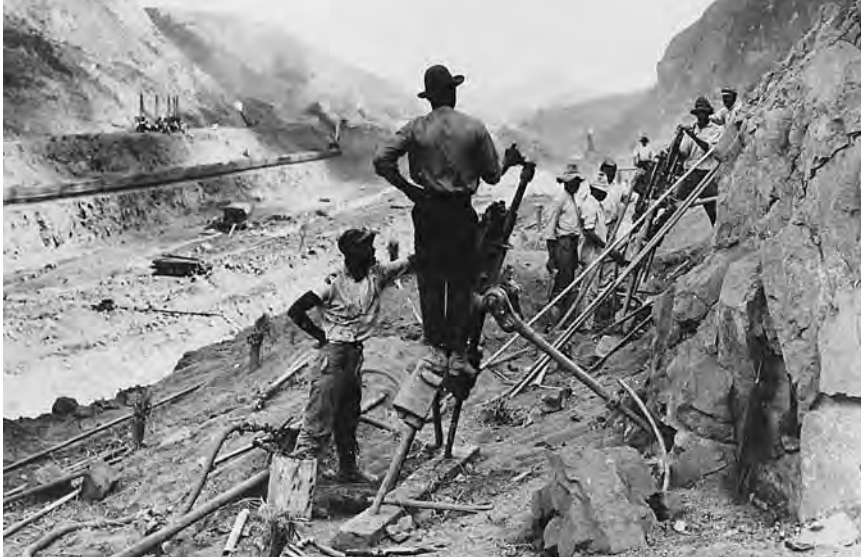
Drilling at Culebra Cut, January 1912 U.S. Military Academy Library
