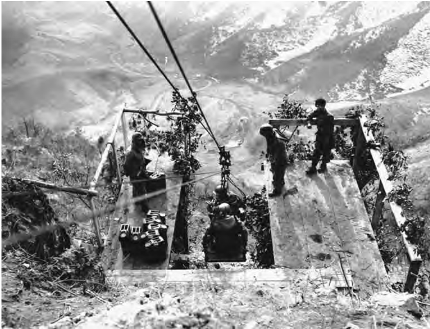
A cable car built by the 3d Engineers carries men and supplies up the steep hillsides National Archives
