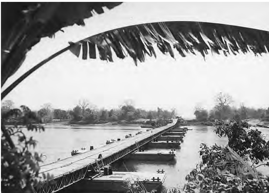
Steel barge bridge along the Ledo Road
