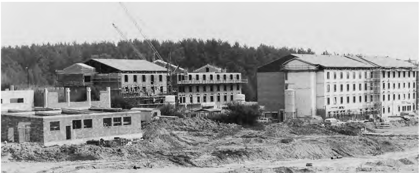
Barracks under construction, Vilseck, West Germany, 1983
