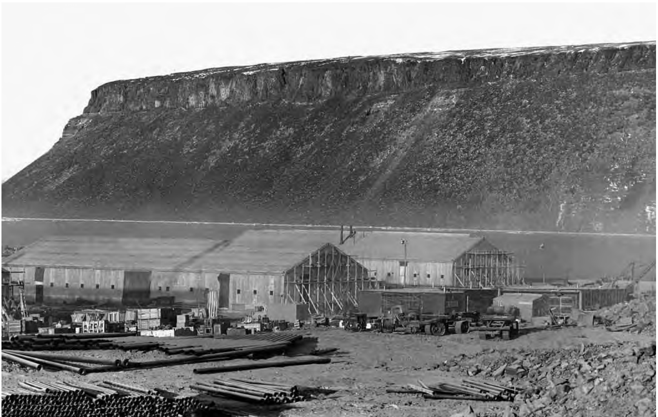
Buildings constructed by the Corps on Greenland to support Project Blue-Jay, October 1951. Project Blue-Jay involved the construction of Thule Air Force Base.
