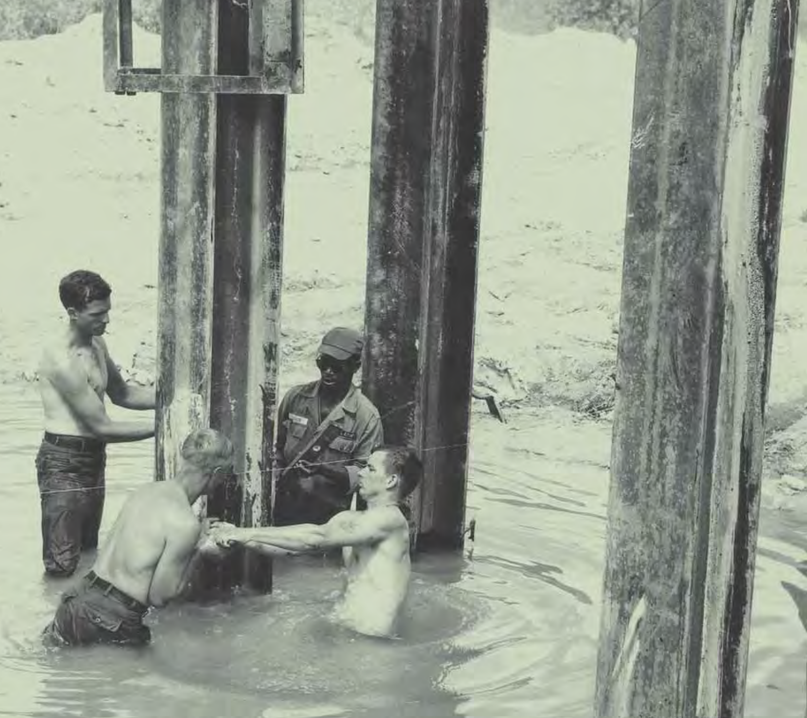
Soldiers of the 299th Engineer Battalion check the alignment of piles before they are driven, May 1966.
