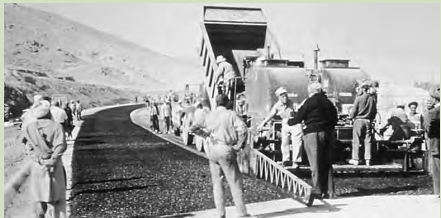
Laying highway asphalt along the ring road
