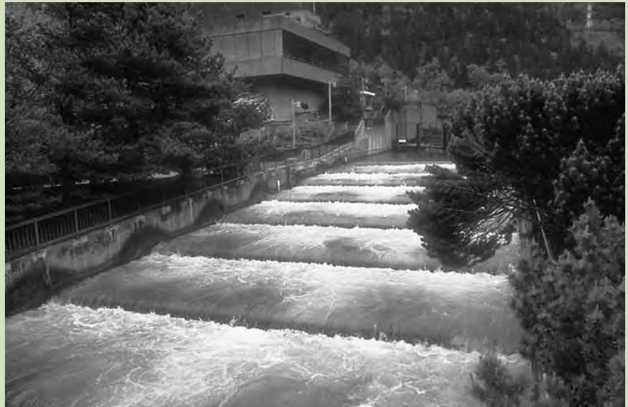
Fish ladder and the Visitors Center at Bonneville Dam, Ore.
