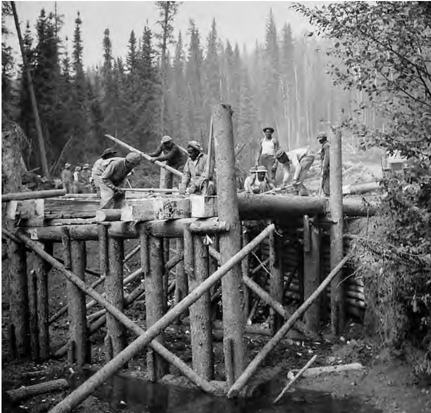
Soldiers of the 95th Engineer General Service Regiment, an African-American unit, building a bridge on the Alaska-Canada (ALCAN) Highway.
