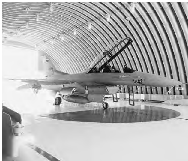
Hardened aircraft shelter with an F-16D completed by the Transatlantic Programs Center at Gianaklis Airbase, Egypt, 1996.
