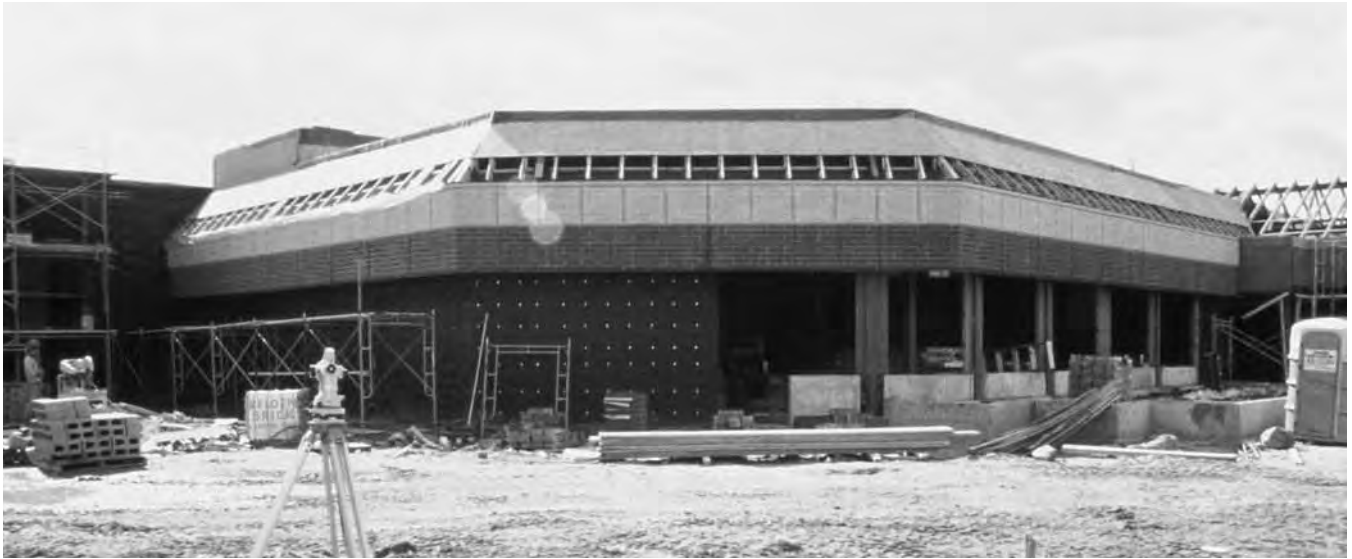
Shopping center under construction at Fort Drum, N.Y.
