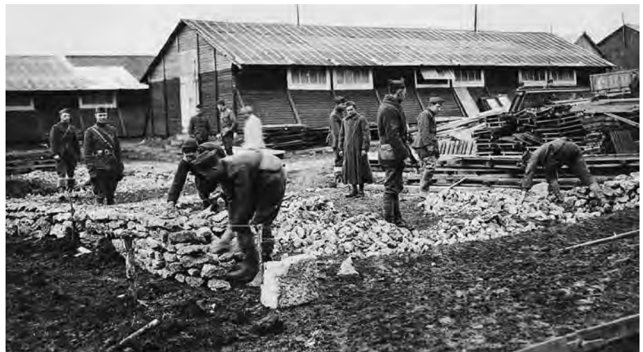
Engineers laying foundation for barracks and hospital in France
