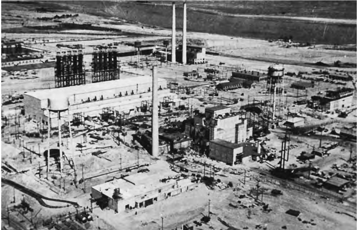
First reactor pile area at Hanford Engineer Works
