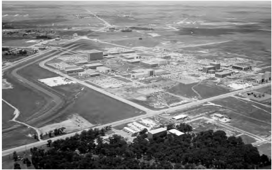
The Manned Spacecraft Center, Houston, Texas, under construction, December 1966.
