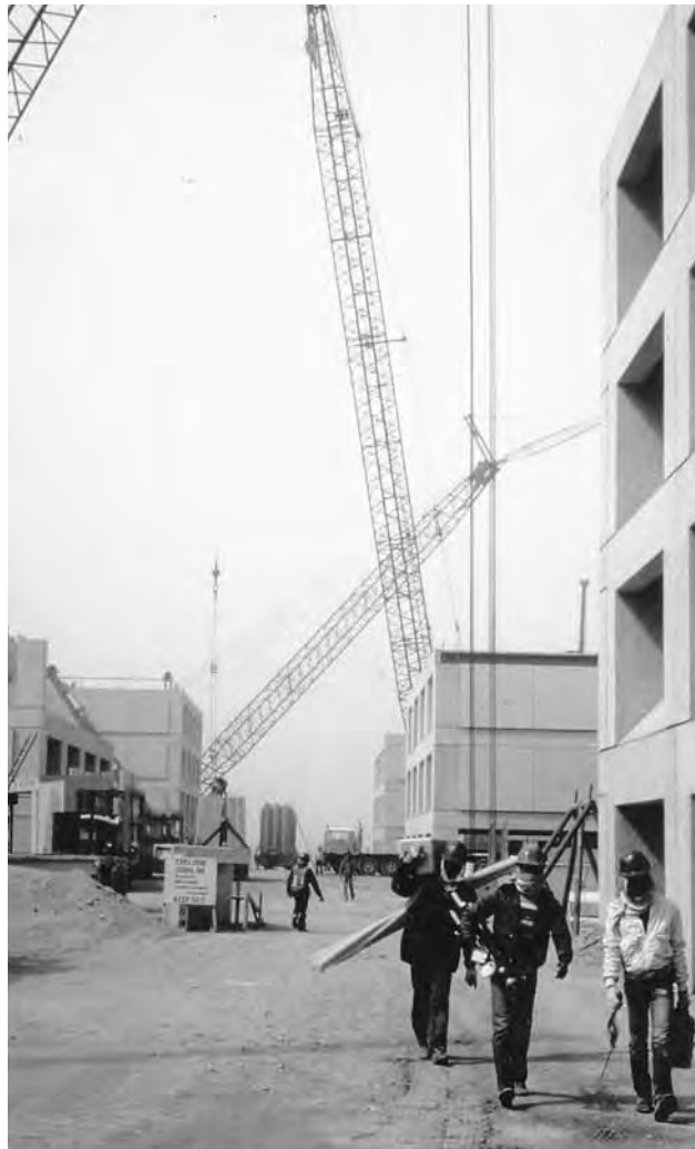
Construction of enlisted quarters, King Khalid Military City, Saudi Arabia
