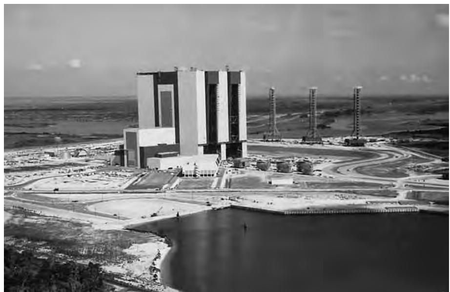
The Vehicle Assembly Building at the Kennedy Space Center. Components for the Saturn V launch vehicle arrived by barge in the basin (foreground).
