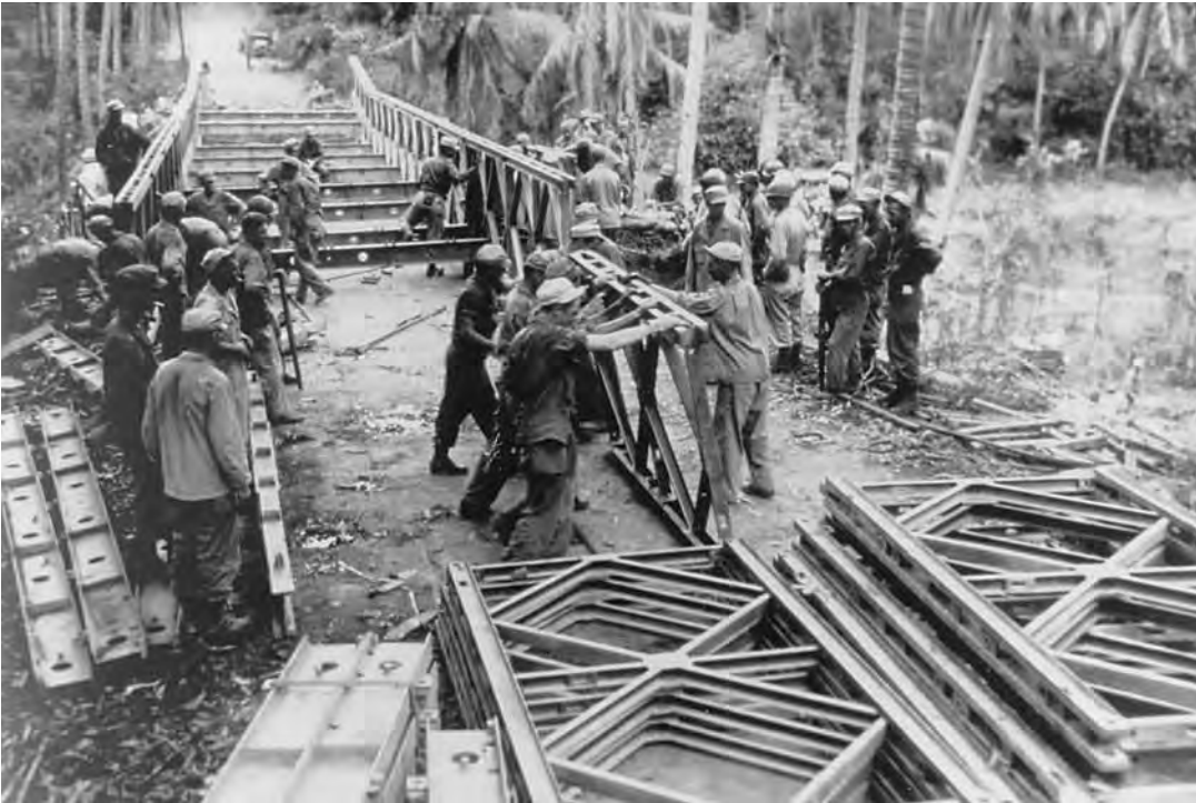
Building a Bailey bridge, the Philippines, 1945
