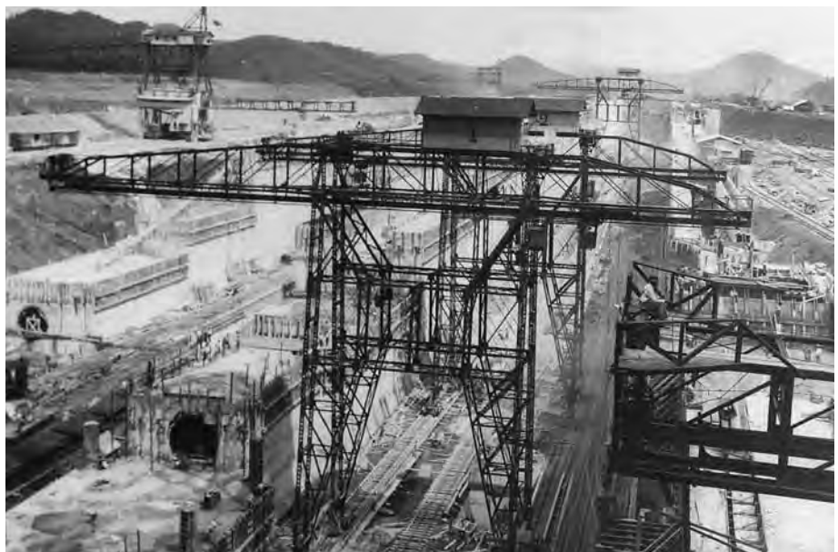
Miraflores Locks under construction, August 1912
