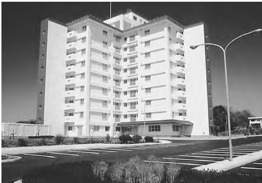
Exterior view of Camp Zama, Japan, high rise family housing, 1999
