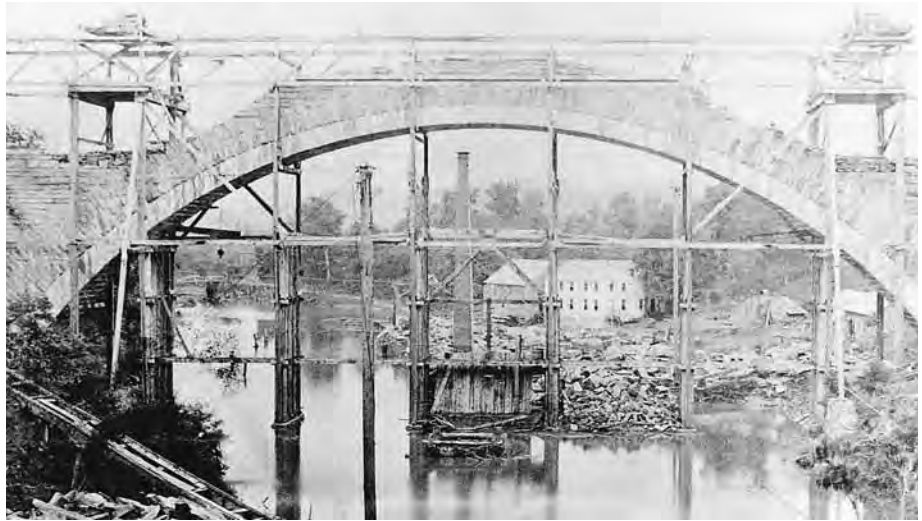
Arch of the Cabin John Bridge under construction, August 12, 1861
