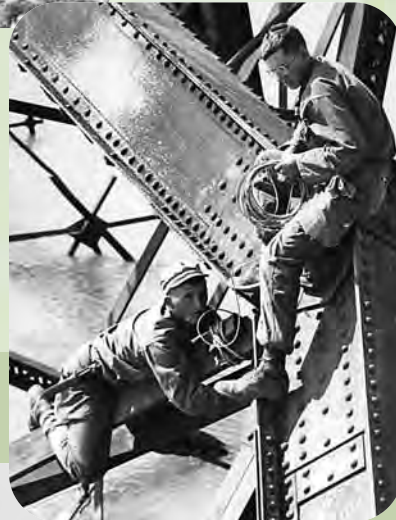
Engineers prepare a bridge for demolition in Korea National Archives
