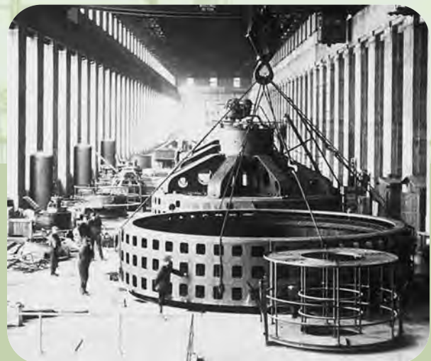
The power generators at Wilson Dam, Tenn., under construction, 1926
