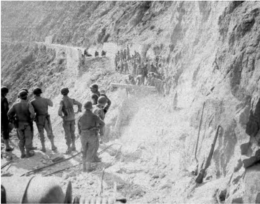
(above) Lacking Bailey bridging equipment, the 10th Engineer Combat Battalion "hung a bridge in the sky" using captured timbers to cross this gap in the road at Cape Calava, Sicily, August 1943.
