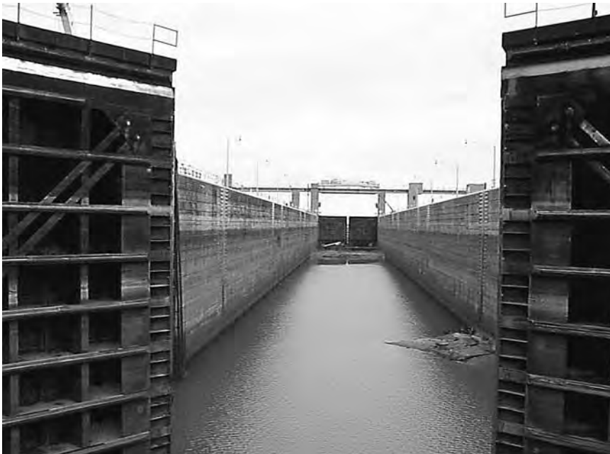
John T. Myers Lock and Dam, Ky.
