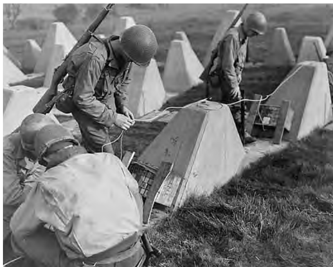
Placing explosive charges to demolish concrete tank barriers on the Siegfried Line, October 1944
