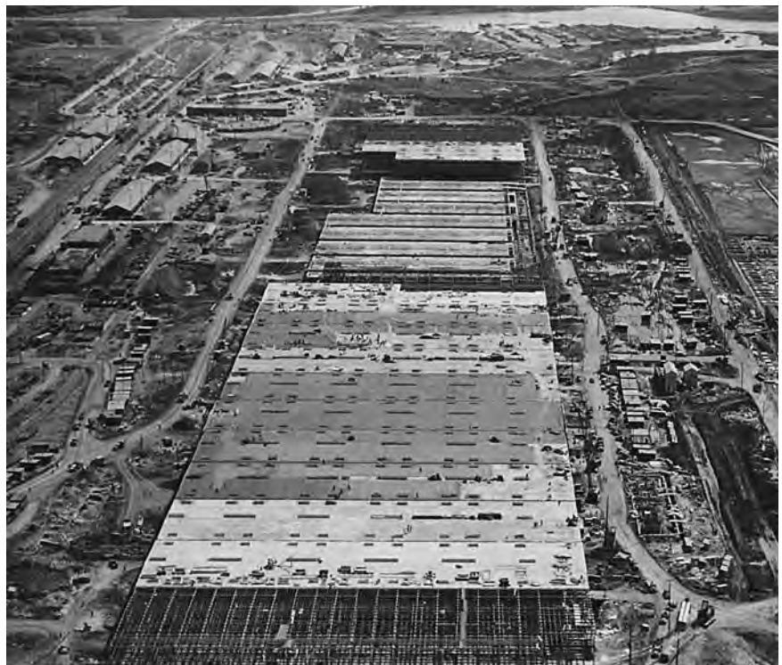
Plant under construction at Oak Ridge, Tenn., April 22, 1944
