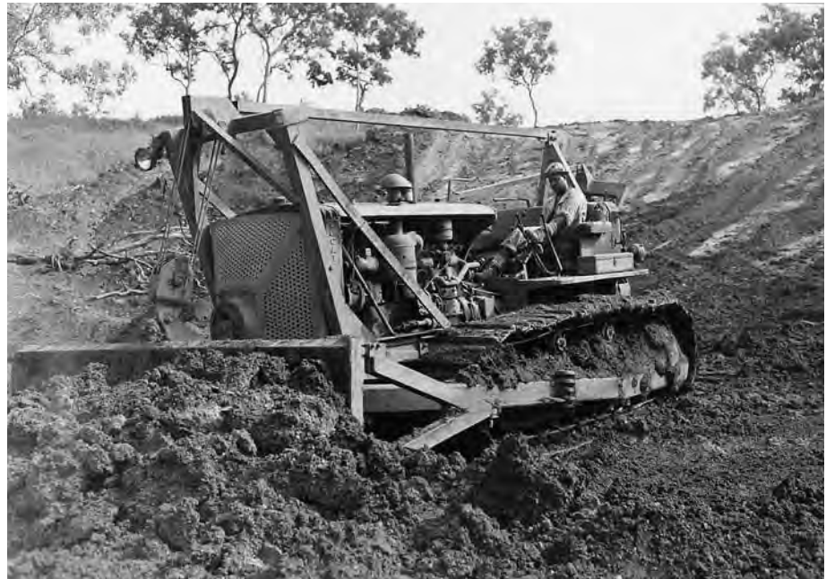
An engineer soldier of the 96th Engineer Battalion, an African-American unit, operating a bulldozer to construct a reservoir near Port Moresby, New Guinea, February 1943.
