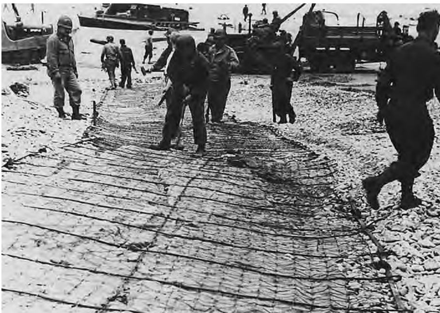
American engineers lay out roads on a French beach, 1944
