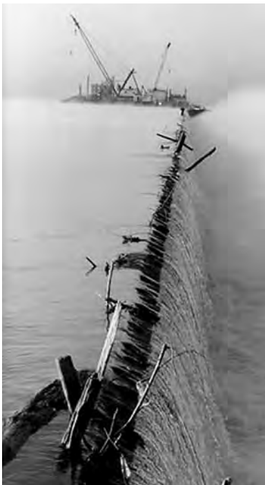
Wicket dam at Lock and Dam 52 on the Ohio River, 1996
