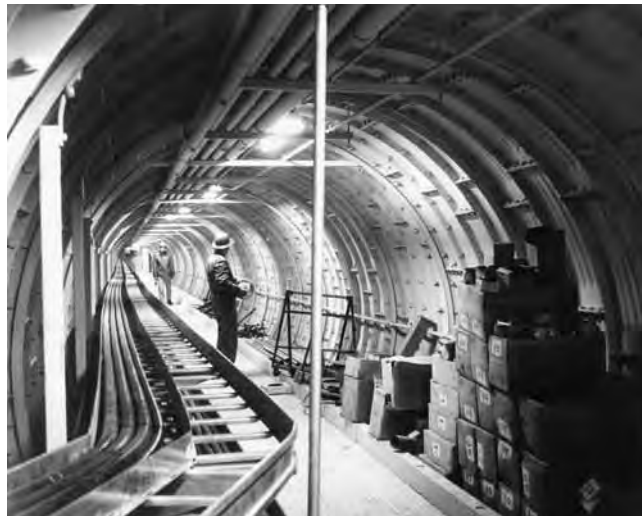
The main tunnel of a Titan I launch complex nearing completion, 1960
