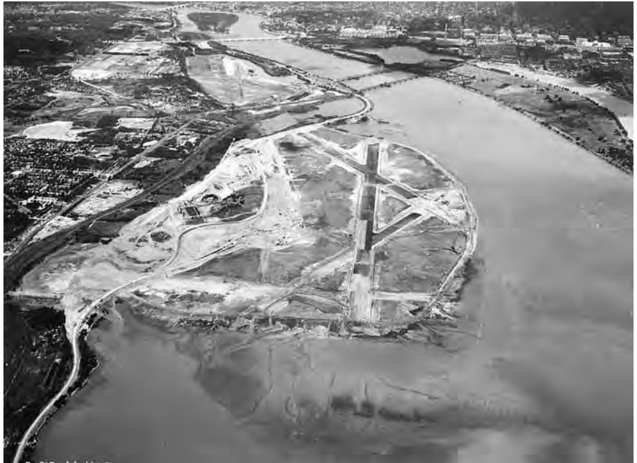
National Airport under construction, July 1, 1940
