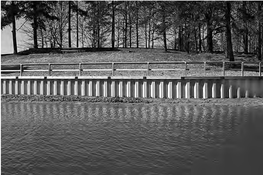
Lake Lanier metal basket erosion control, Buford, Ga.
