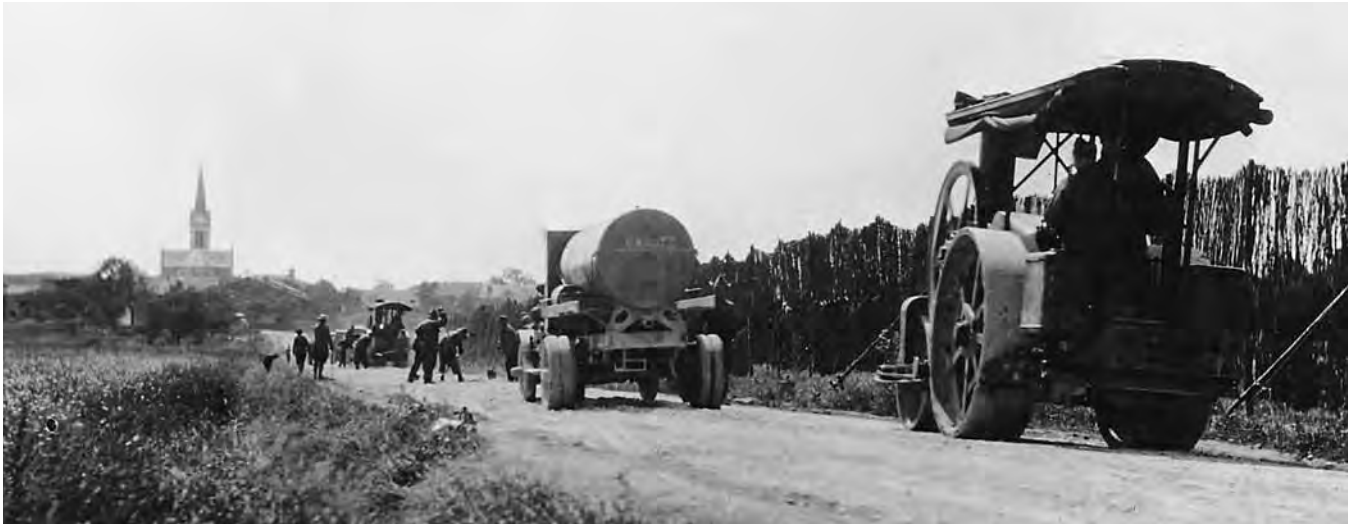
Road construction, France
