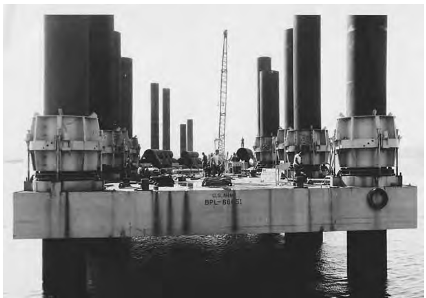
DeLong pier floated into position with caissons ready to be driven down, Cam Ranh Bay, December 1965.
