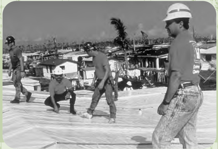
Installing temporary roofs following Hurricane Andrew
