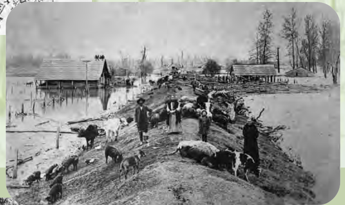
During a 1912 flood, residents of Hickman, Ky., find refuge on levees and rooftops.
