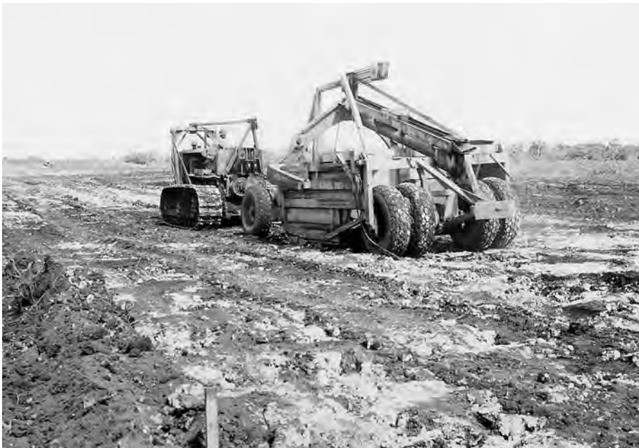
Engineer aviation battalions used heavy equipment such as bulldozers and carryalls to construct airfields for heavy bombers, Kiriwina Island, July 1943.
