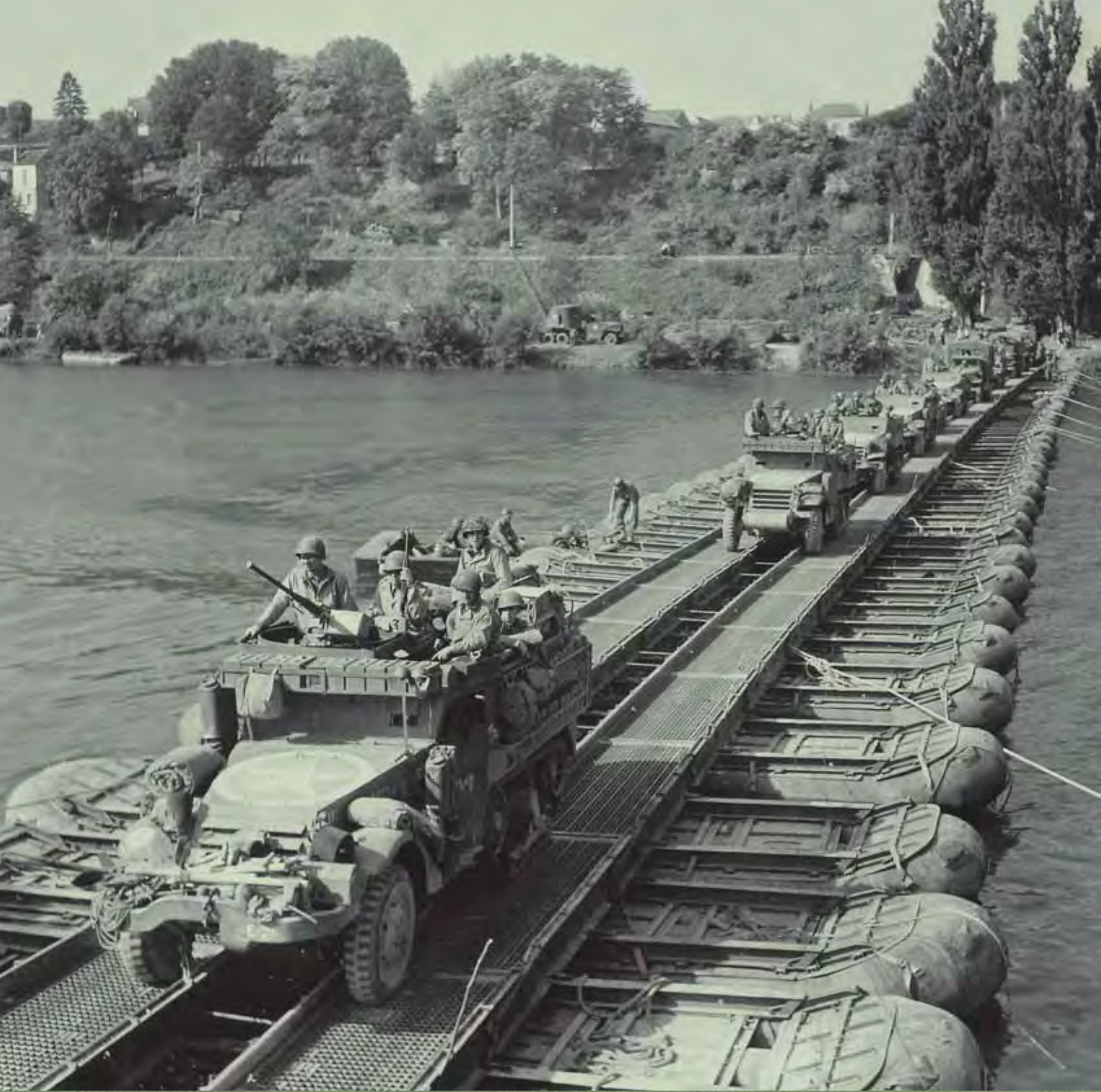
Vehicles of the 3rd Armored Division cross the Seine River on an engineer-built ponton bridge, August 1944
