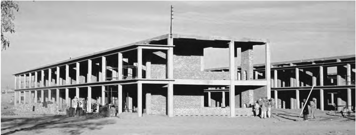
The Corps built a cantonment for the Pakistani army at Multan to accommodate 8,500 troops. The barracks above were two structures of the 310 built on the post. Construction at Multan began in 1959 and was complete two years later.
