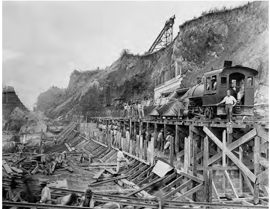
A rail line assisted the canal's construction.
