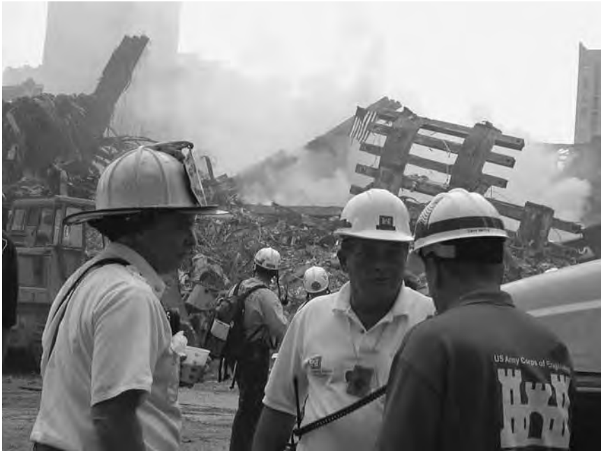
Corps of Engineers personnel confer with a member of the New York City Fire Department at the World Trade Center, September 2001.
