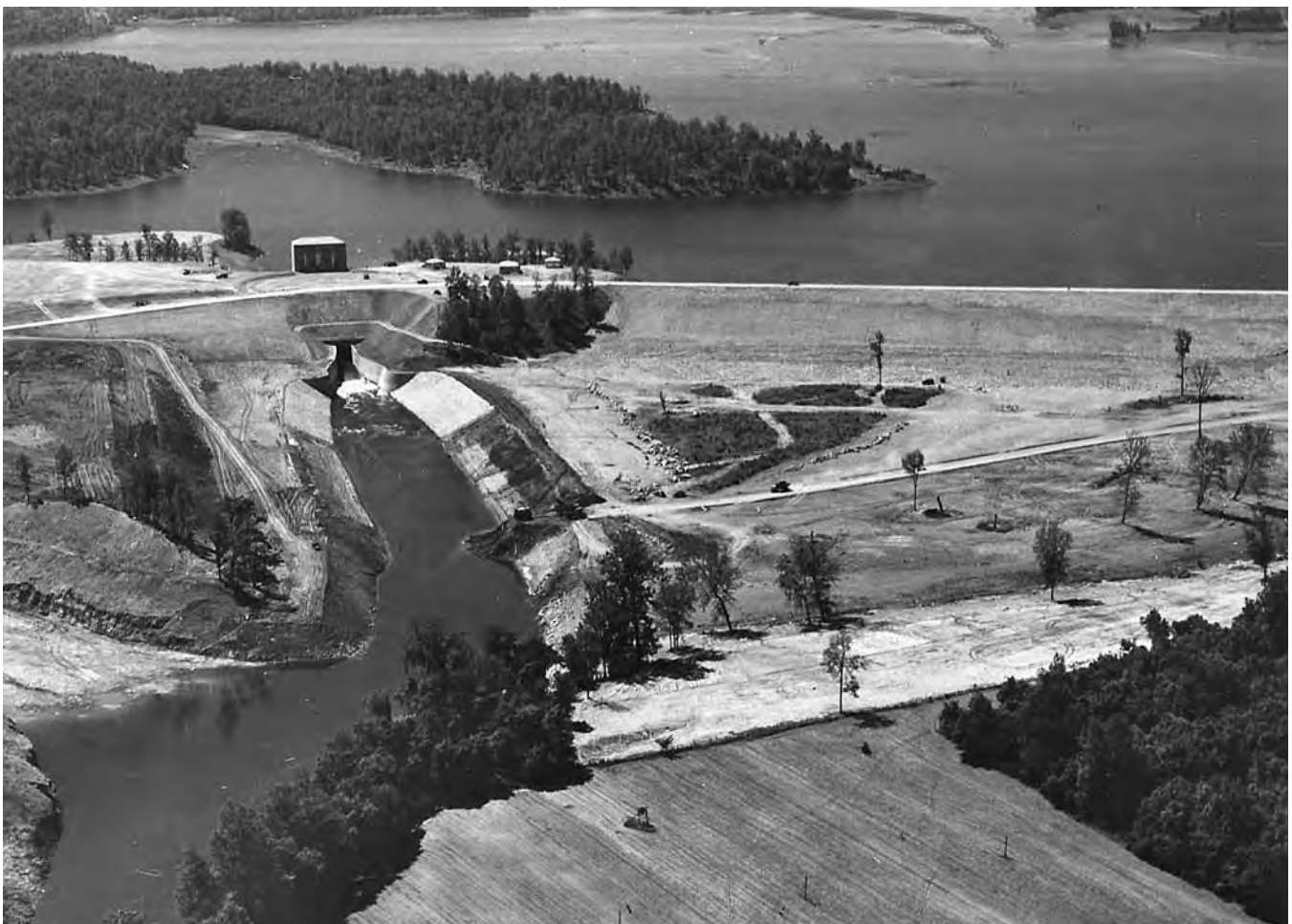
Wappapello Dam on the St. Francis River, Mo., 1941. Wappapello is a vital component of the flood control system for the Lower Mississippi River.
