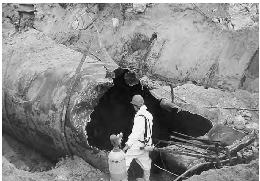
Preparing to remove underground storage tank at the former Kincheloe Air Force Base, Kinross, Mich., 1994
