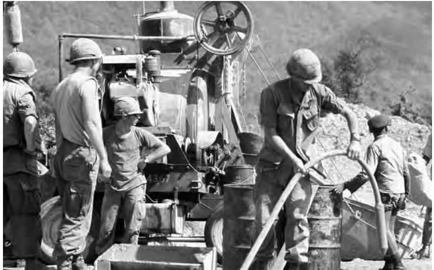
Engineers pour concrete for a new bridge approach.
