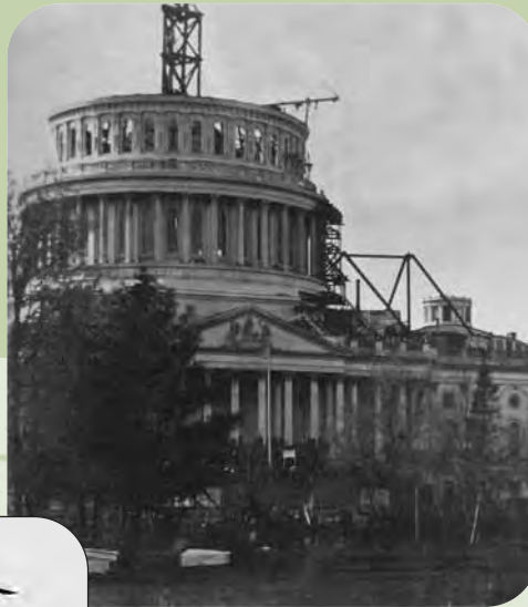
Capitol dome under construction, 1861
