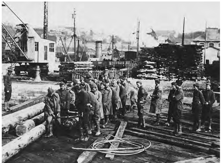
(above) 33rd Engineers carry a thirty-foot section of mast for a stevedore derrick, western France
