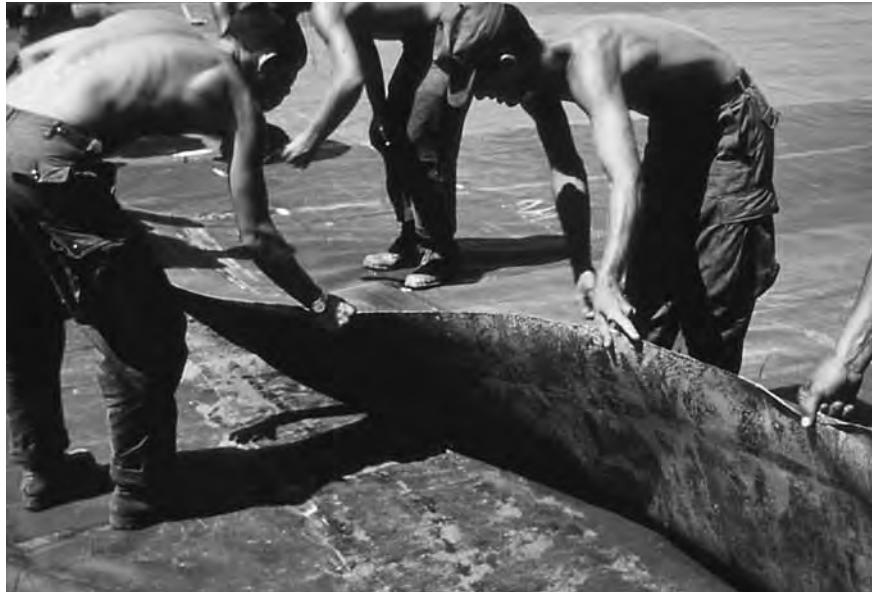
Spreading T-17 membrane on a runway
