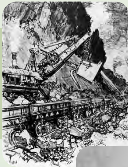
Steam shovel at work in the Culebra Cut; a lithograph in a series on the Panama Canal by Joseph Pennell, noted American artist and illustrator
