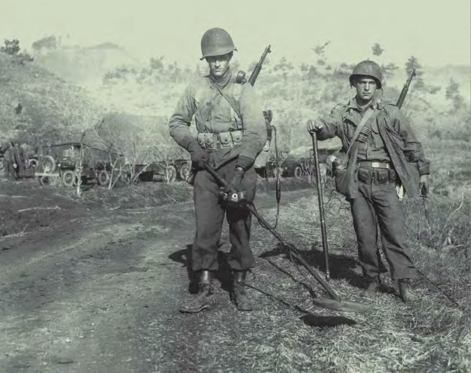
Soldiers of the 2d Engineer Combat Battalion sweep a road for anti-tank mines, March 1953 National Archives
