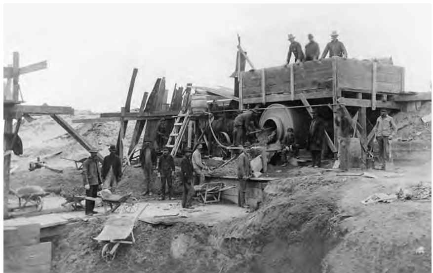
Mixing plant on the Illinois and Mississippi Canal, 1900
