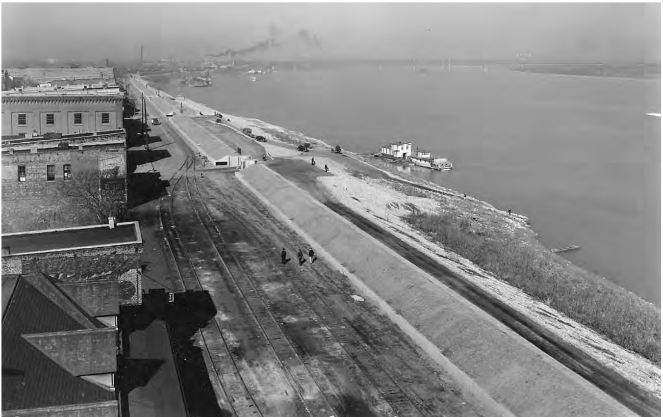
Floodwall at Cairo, Ill., 1936
