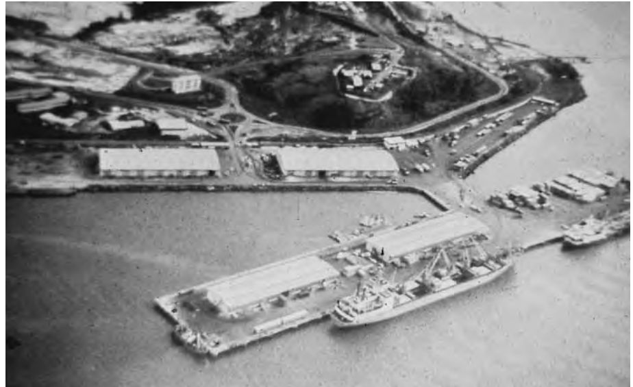
Port of Owendo, Gabon, site of Corps studies undertaken for the Agency for International Development
