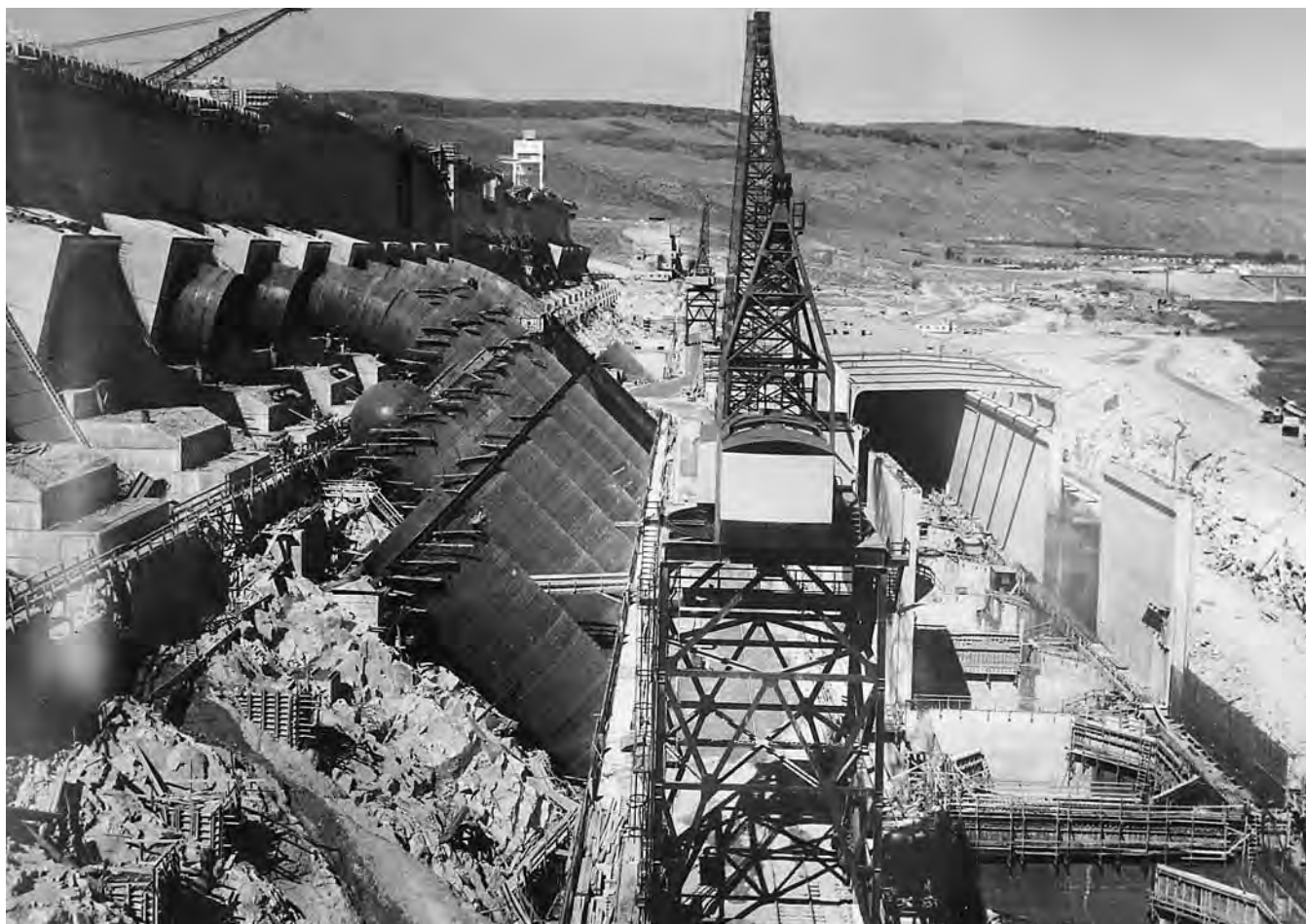
Chief Joseph Dam under construction, Wash., 1955
