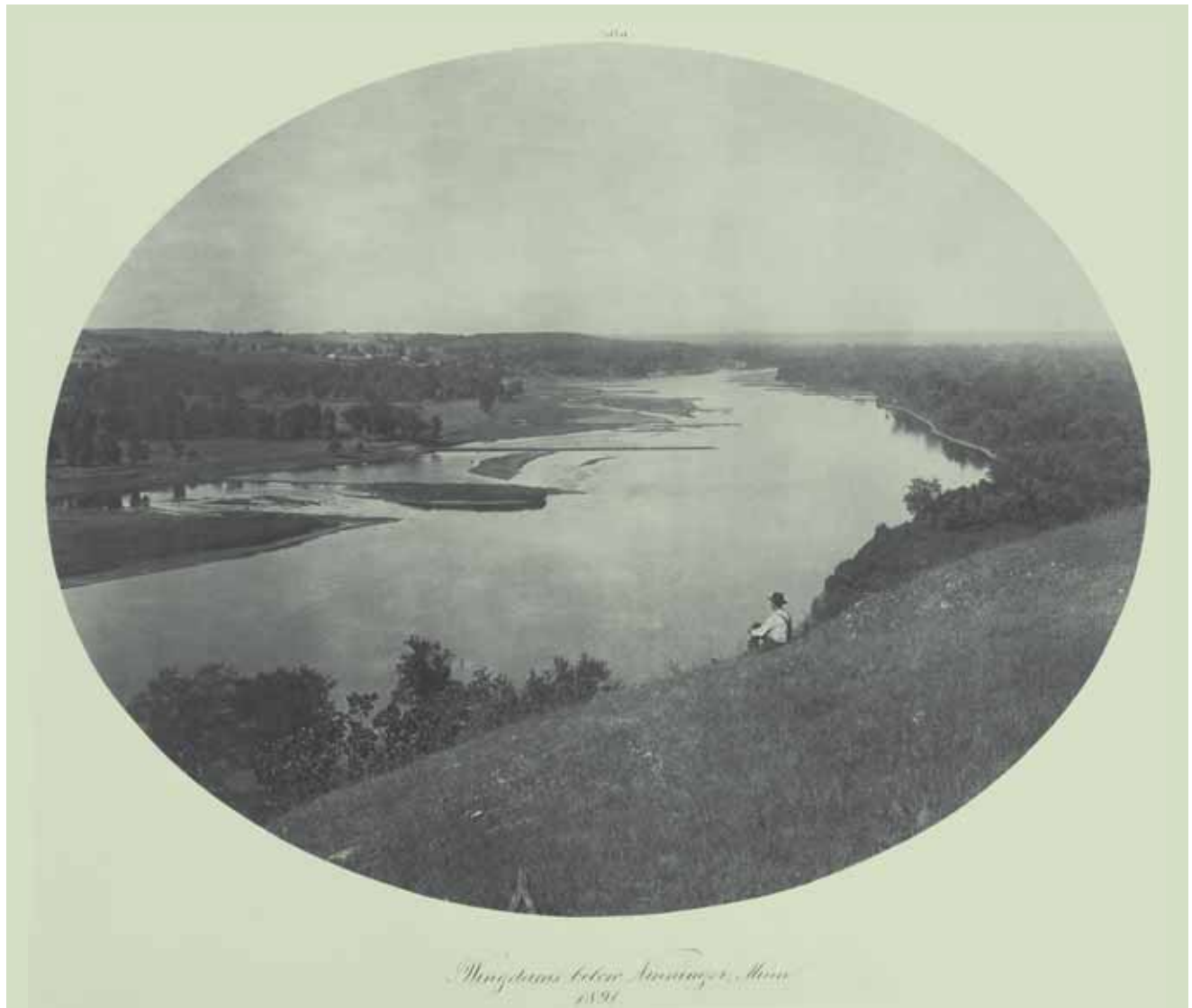
Henry Bosse photo of wing dams below Nininger, Minn., on the Upper Mississippi River in 1891. These river structures were designed to constrict the river at shallow places, resulting in a narrowing and deepening of the channel.
