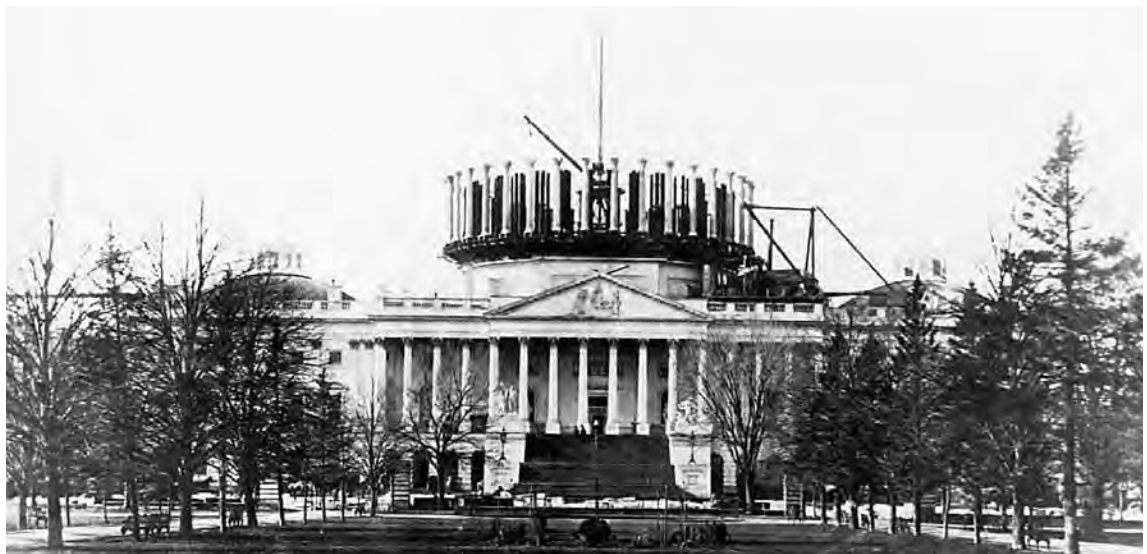
U.S. Capitol dome under construction, December 31, 1857
