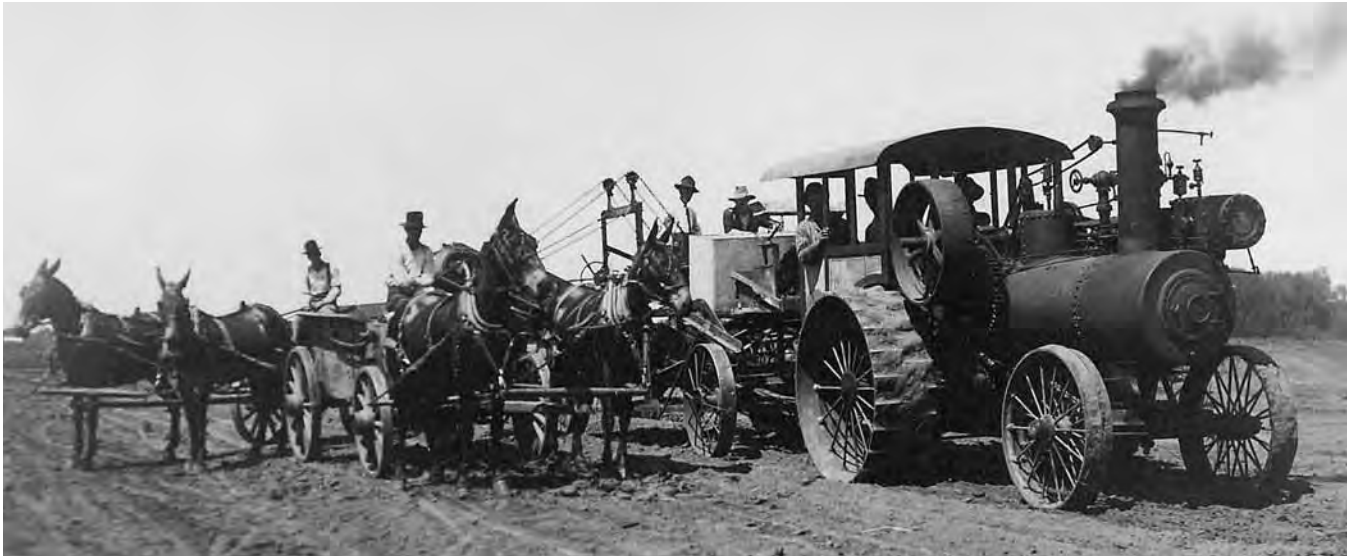
Excavating the Illinois and Mississippi Canal, 1904
