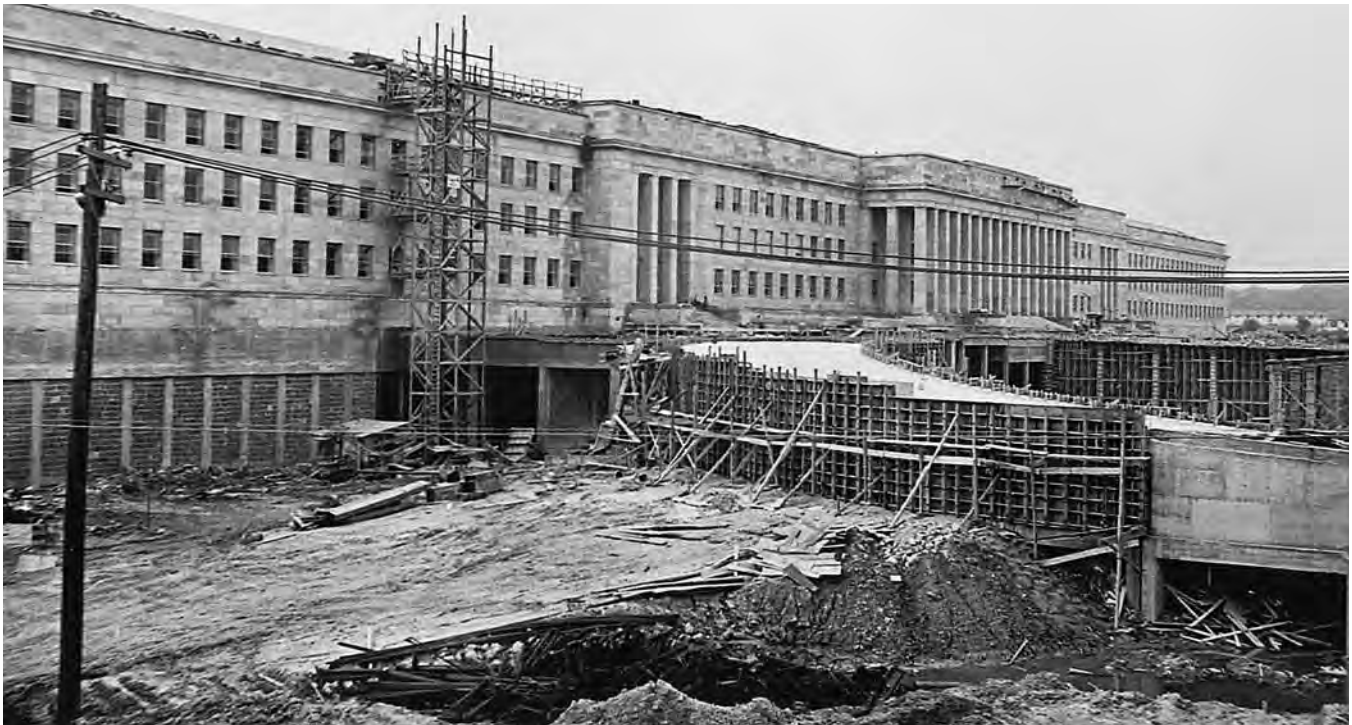
The Pentagon under construction
