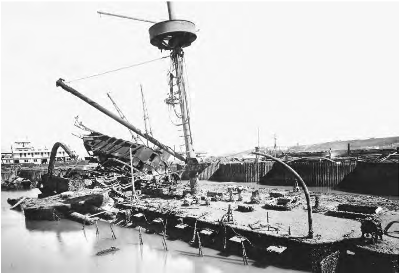
The sinking of the U.S.S. Maine in 1898 inflamed public opinion and pushed the U.S. into war with Spain. After the Spanish-American War, the Corps of Engineers built caissons in 1911 around the Maine in Havana harbor and pumped out water so the ship could be examined before it was towed to deep water and sunk in its final resting place. The USACE Museum Collection has the Maine's ship's wheel that the Corps received in appreciation for its work in raising the famous ship.
