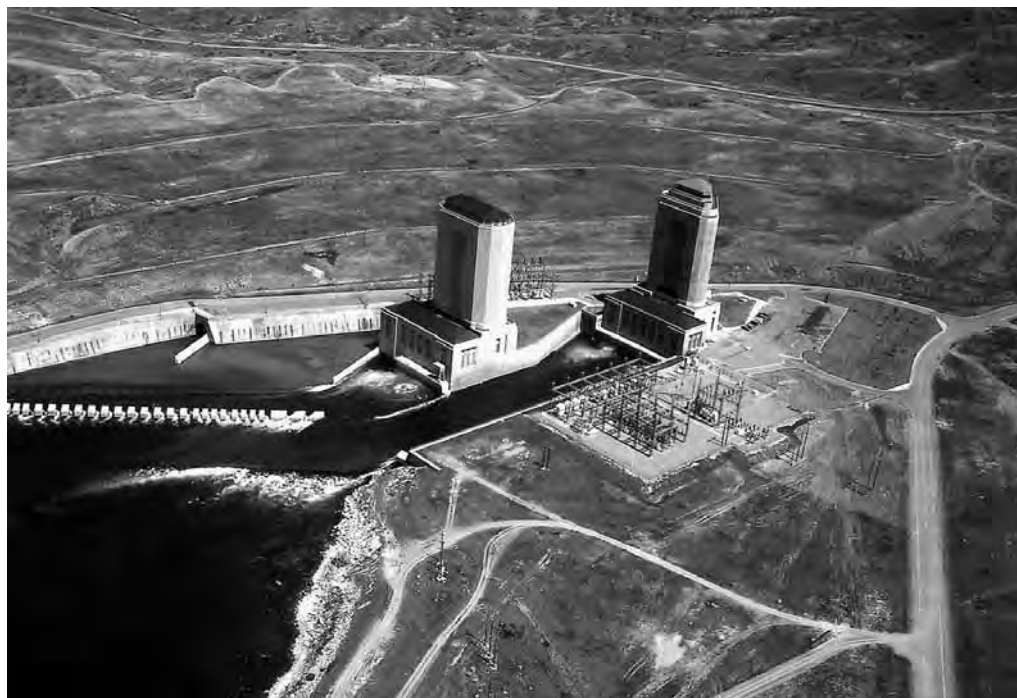
Powerhouses, surge tanks, and switchyard at the Fort Peck Dam along the Missouri River, Mont.
