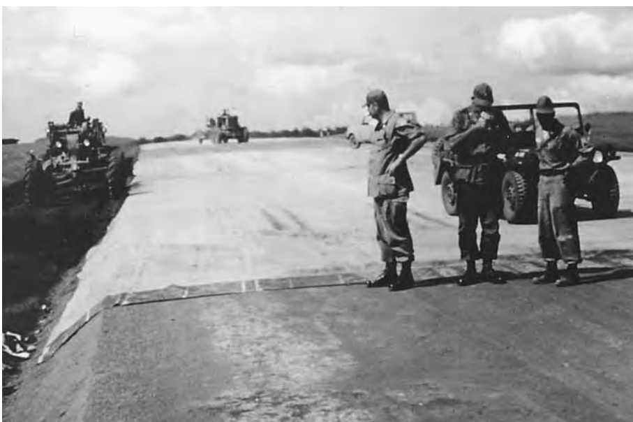
Installing T-17 membrane at Bao Loc Department of Defense
