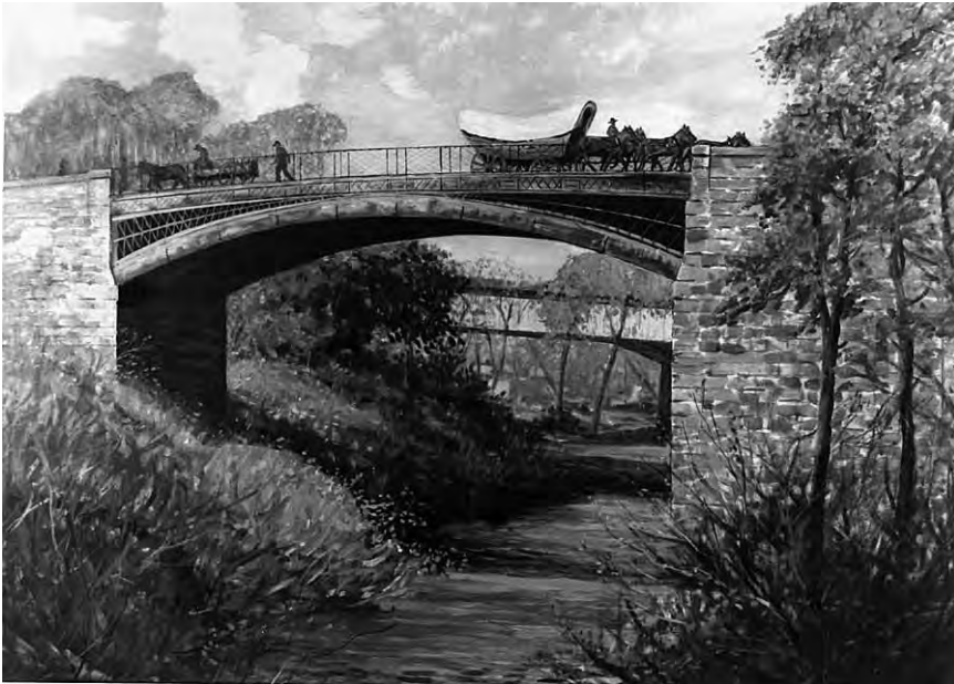
First cast-iron arch bridge built in the United States. Carl Rakeman painted this image of the Dunlap Creek Bridge.
