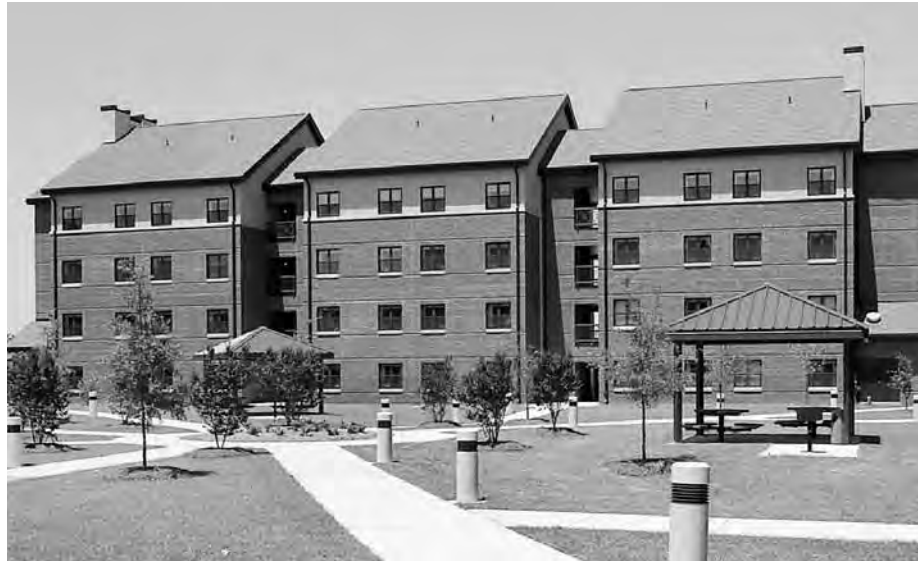
Barracks at Fort Bragg, N.C., 2003
