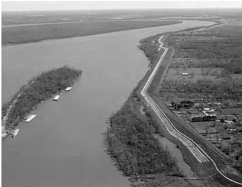
A flood control levee just below Medora Crossing on the Mississippi River at Mile 210
