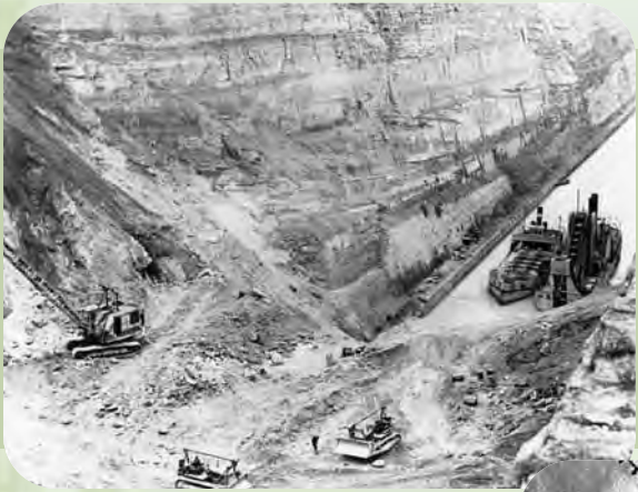
The dredge Poseidon clearing the Corinth Canal in Greece, 1947
