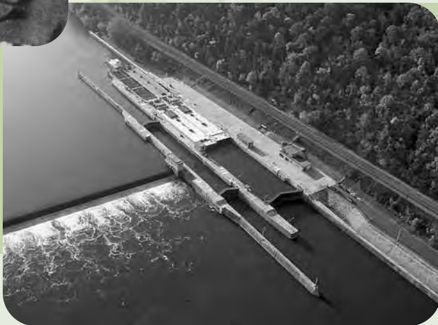
Dashields Locks and Dam on the Ohio River near Glenwillard, Pa., opened for navigation August 1929.
