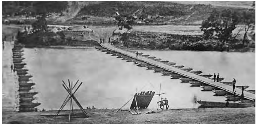
Ponton bridges across the Rappahannock River built by 50th and 15th New York Engineers, 1863.
