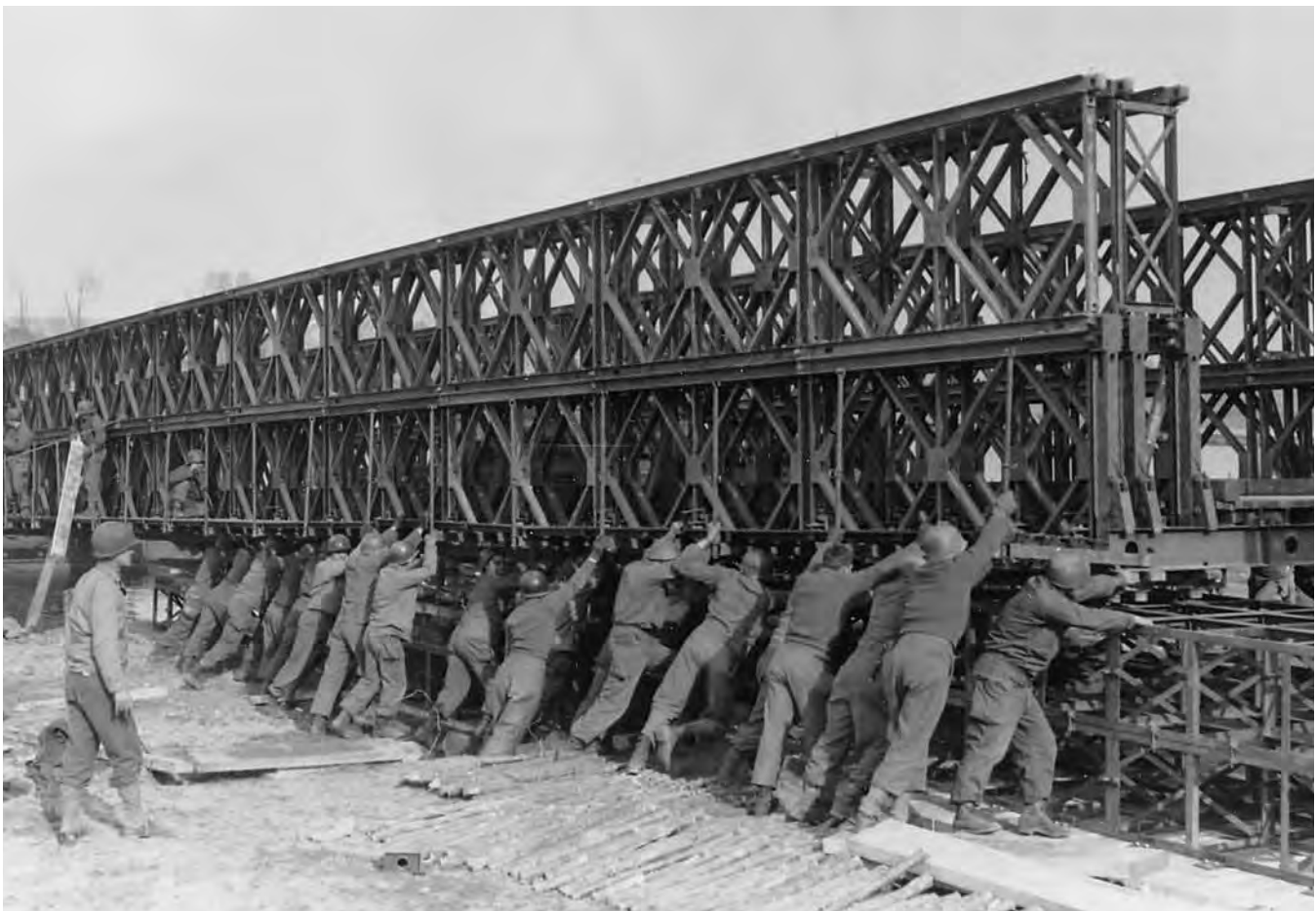
Engineers assembling a Bailey bridge to put across the Rhine River at Wesel, March 1945
