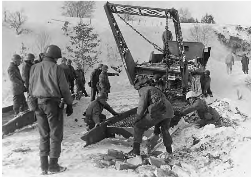
Assembling a treadway bridge in Belgium, 1945
