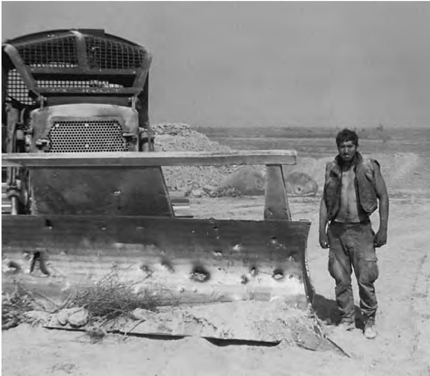
60th Land Clearing Company's Rome plow
