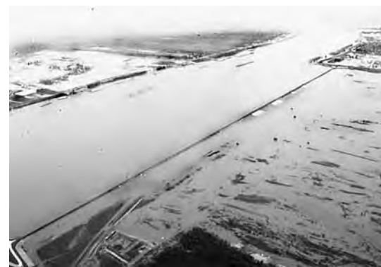
Floodwater over Bonnet Carré Spillway
