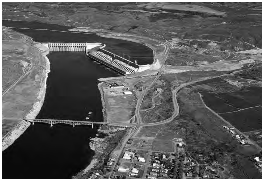
Contemporary view of Chief Joseph Dam along the Upper Columbia Basin
