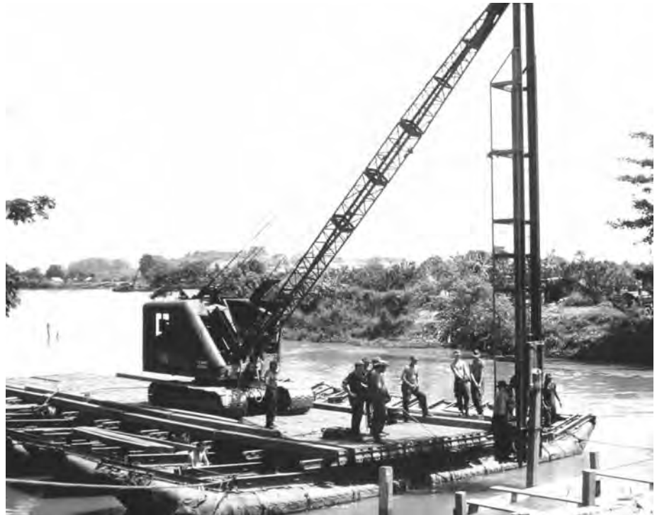
Soldiers of the 1st Engineer Battalion driving pile for the construction of a new bridge near Di An
