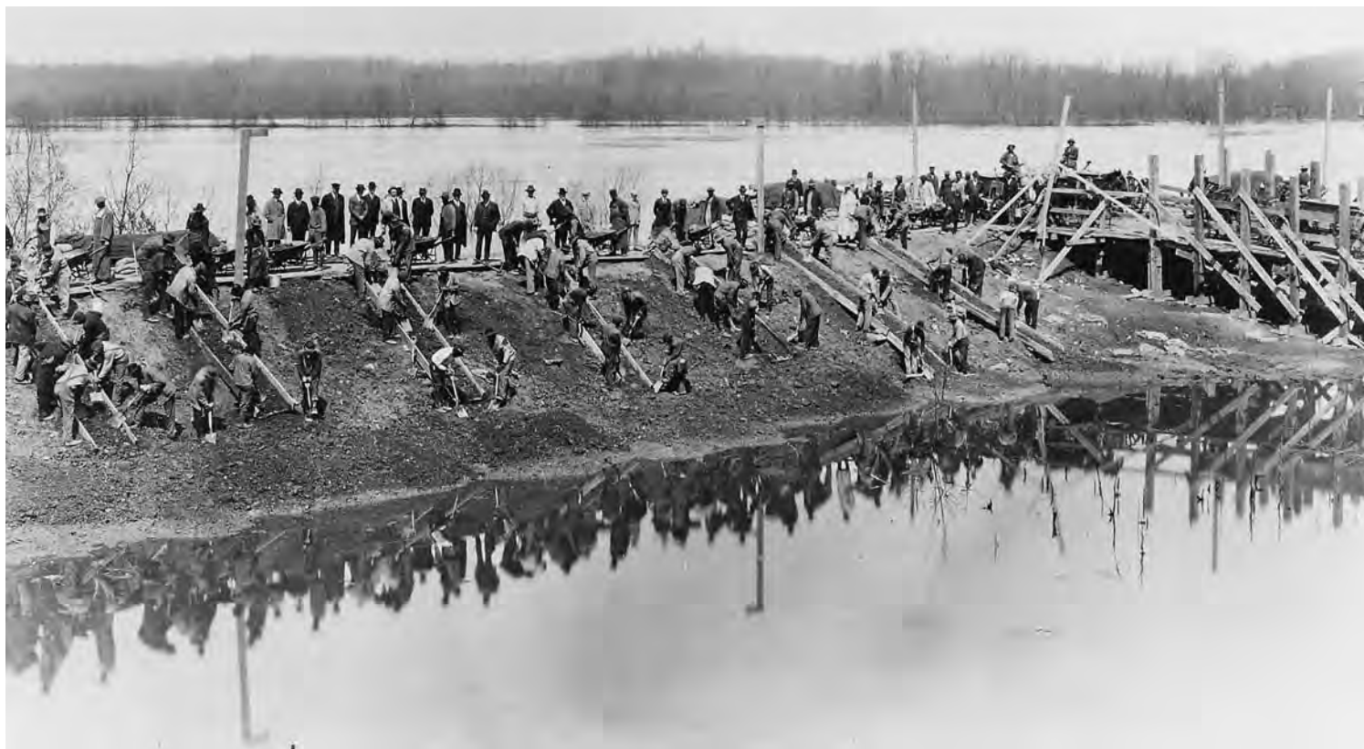
Shoring up a levee near Memphis, Tenn., 1927
