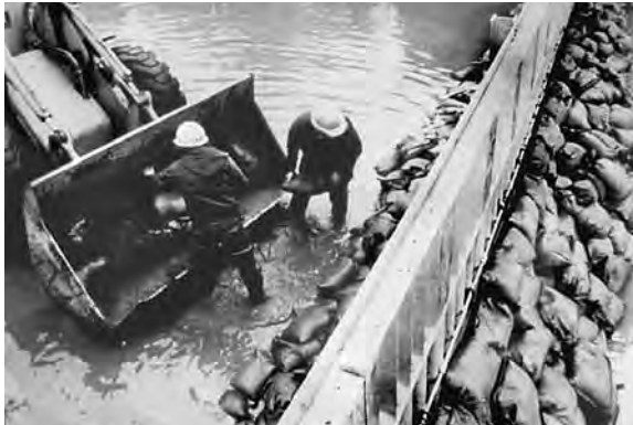
Corps personnel laying down sandbags
