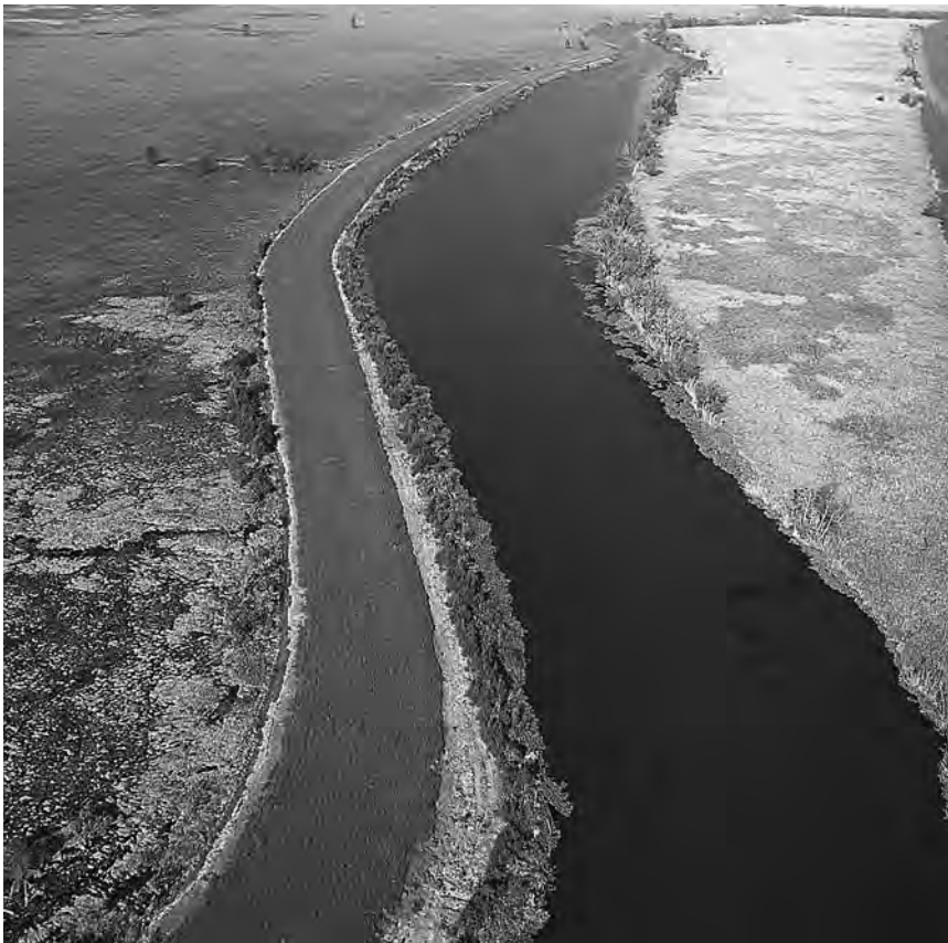
Davis Pond Freshwater Diversion Project: lower guide levee at Lake Salvadore at Mile 150 on the Mississippi River, La., 1998
