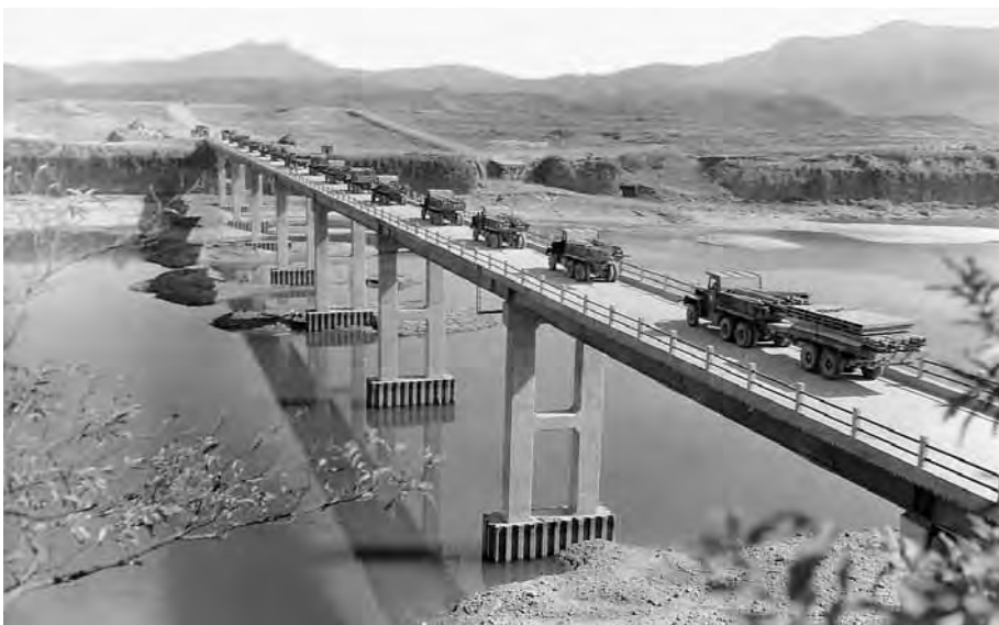
Built by the 84th Engineer Construction Battalion, the Libby Bridge provided a vital high-level crossing of the Imjin River, July 1953.
