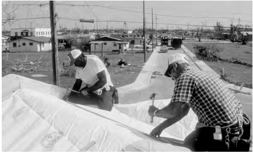
Corps of Engineers contractors install a temporary roof on a home damaged by Hurricane Andrew.
